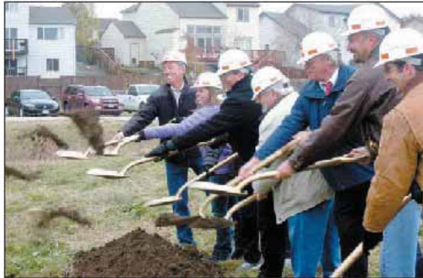
Castle Rock town officials throw the first shovel of dirt at the Oct. 29 groundbreaking ceremony near Castle View High School of a two-mile two-year road project that will extend Meadows Drive to Interstate 25. Photo by Virginia Gantier
